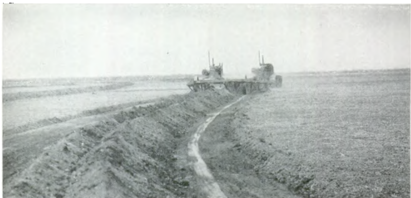
Figure 3.—Constructing levees in a California rice field.
