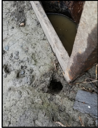
Figure 2. Leak near outlet caused by crayfish.
